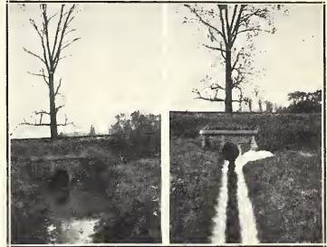
FIG. 3. Artesia, Mississippi. Left, before malarial control drainage; right, after construction of reinforced concrete invert with sodded banks.
